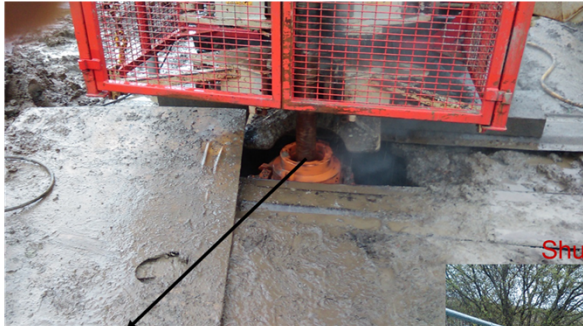
Top of the valve with a drilling rod going through
