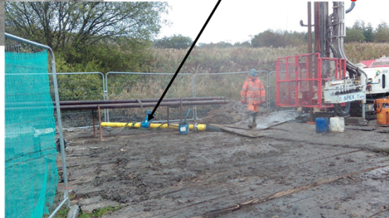
Shut off valve underneath the drilling rods
